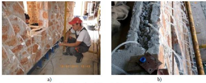
Fig. 5 Grouting of three-leaf masonry walls
