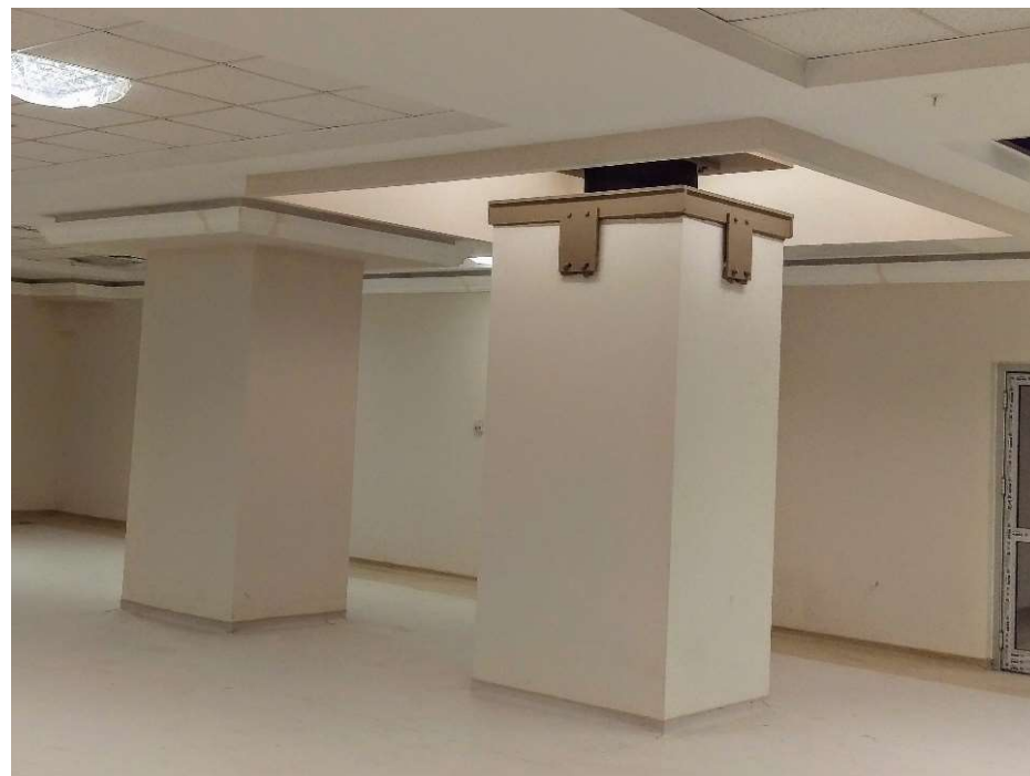
Seismic isolation retrofit application (Photo credits B. Sadan)
