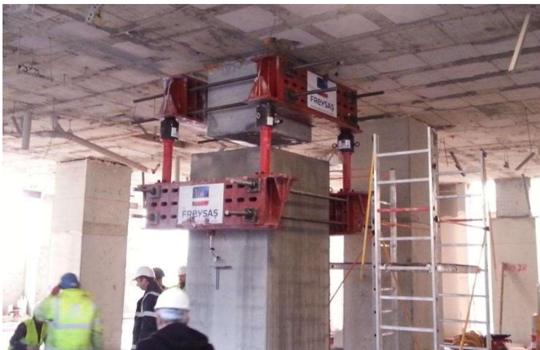
Cutting of the column (Photo credits R. Turan)
