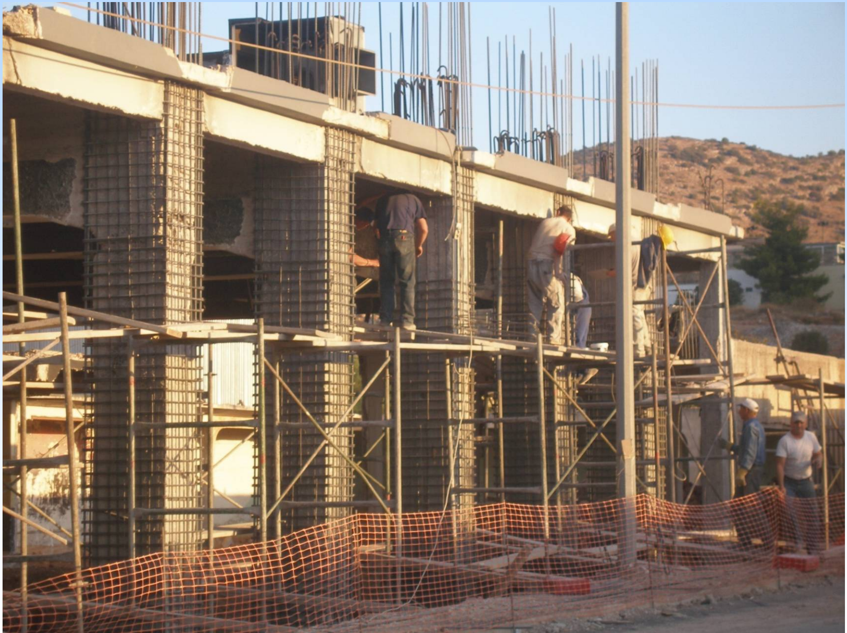
Concrete jacketing in practice
