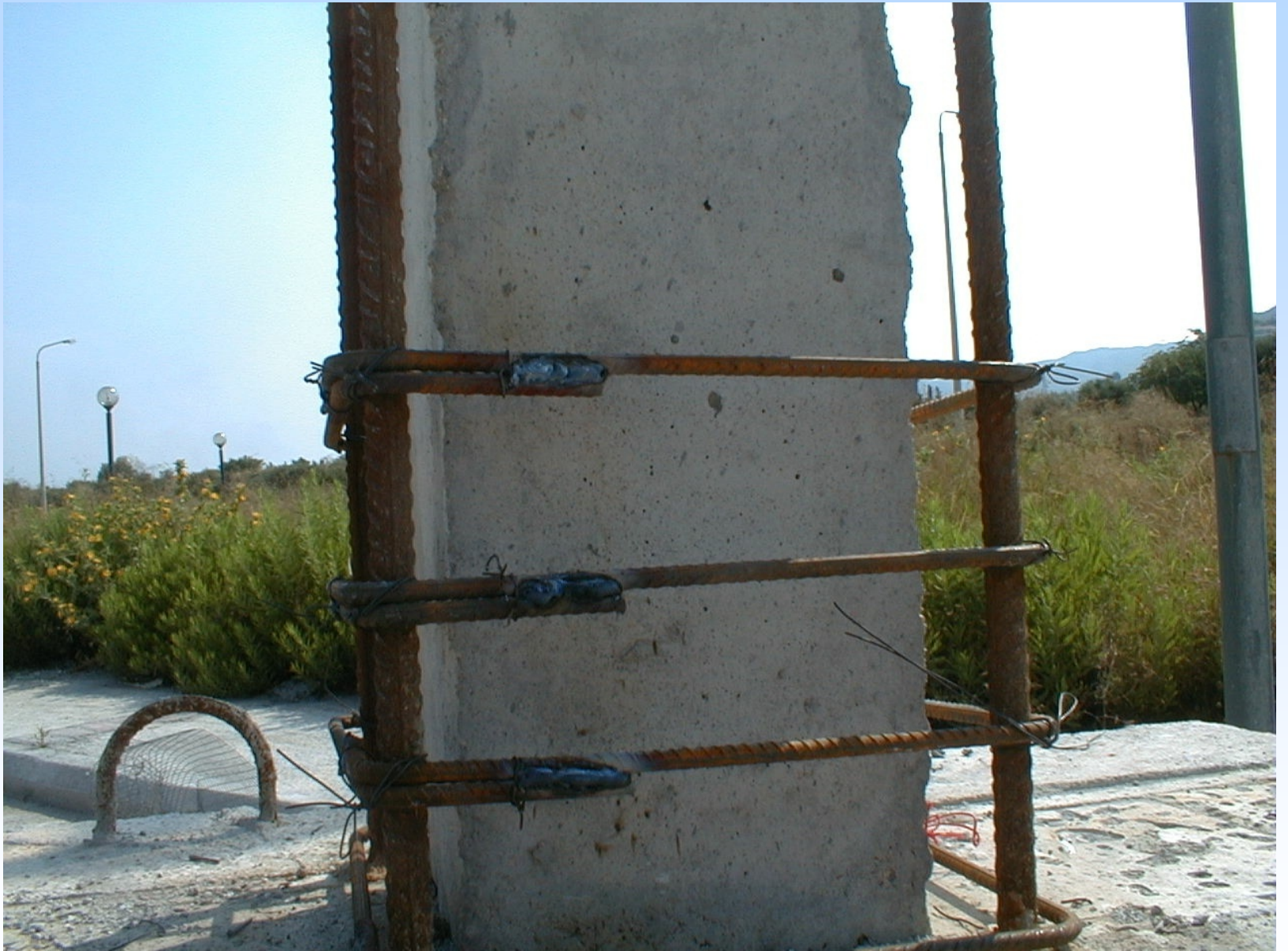
Welding of jacket's stirrup ends
