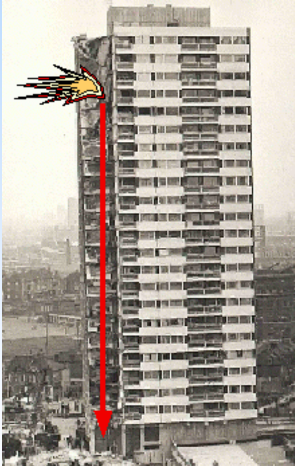
Ronan Point (London 1968) Gas explosion on 18 th floor
