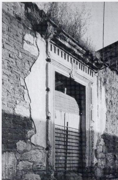
Figure 8.6 Mexico. Failure of the cement capping, cracked by thermal movement, has opened the way to the detachment of the rigid sheathing of the mud block core (r.h.s.).
