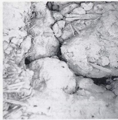
Figure 8.11 A circumstance where structural elements of a predominantly earth wall are in contact. The introduction of a plastic fill stage by stage would be considered here (courtesy of Rebecca Warren).
