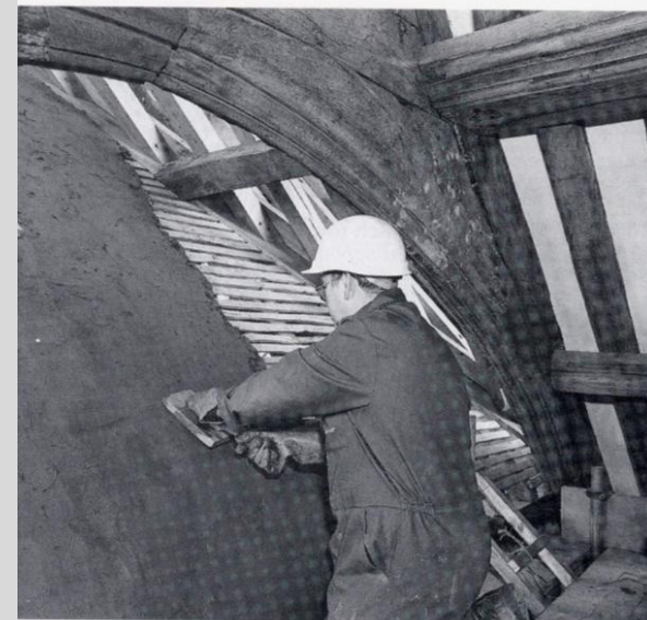
Figure 9.3 Bowhill: Great hall ceiling/Great chamber – applying daub and scat (© English Heritage)
