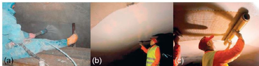
(a) Surface preparation by hydrojetting; (b) application of the inorganic matrix; and (c) application of the PBO textile reinforcement. Kind permission of Ruredil SPA.
