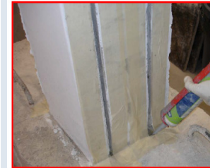
Grooves and holes were filled by injecting the bonding agent
