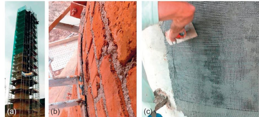
The unreinforced masonry chimney: (a) with scaffolding during repair; (b) before strengthening; and (c) during strengthening with carbon fiber textile bonded in a cementitious matrix. Kind permission of Ruredil SPA.
