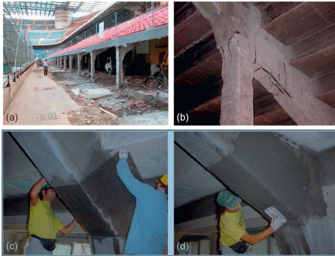
(a) Existing RC frame supporting the tier of seats; (b) typical damage found in RC beams; (c) application of a U-shaped TRM jacket for shear strengthening of the beam; and (d) strengthened beam at the end. Kind permission of Ruredil SPA.
