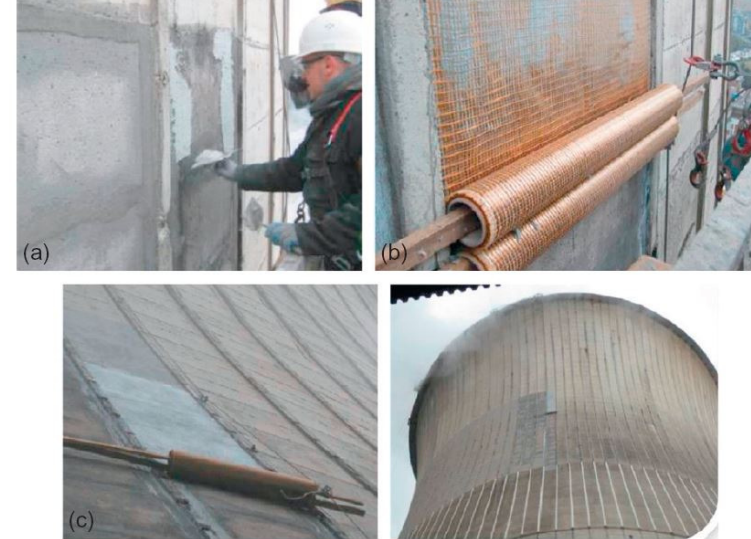
(a) Screeding of the inorganic matrix on the tower shells; (b) application of two layers of PBO textile reinforcement; and (c) overview of the strengthening application. Kind permission of Ruredil SPA.
