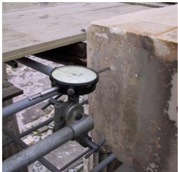
*Monitoring the movement of the columns during the dismantling*
