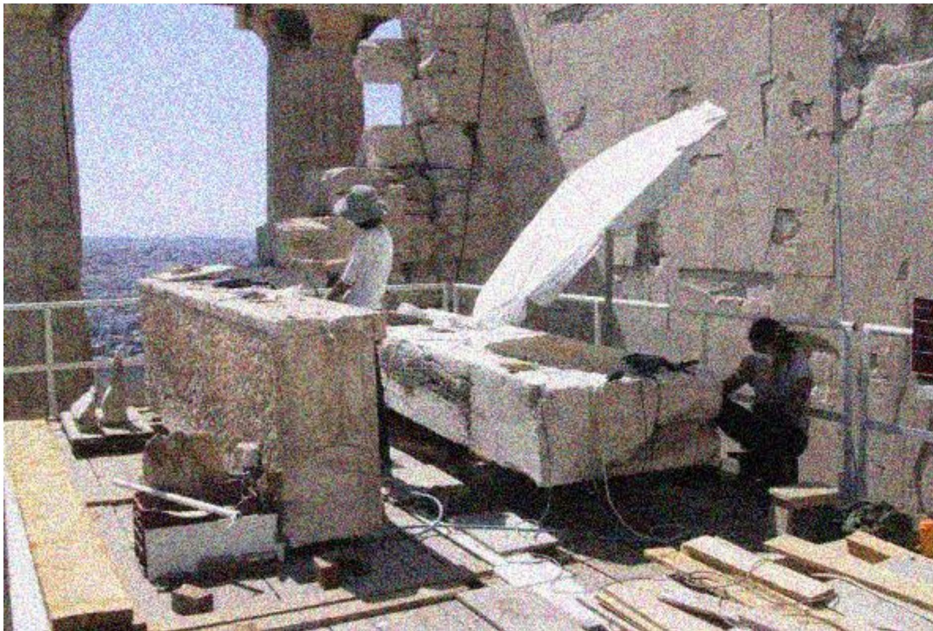
*Removal of all steel clamps and dowels, conservation of the unbroken architraves*
