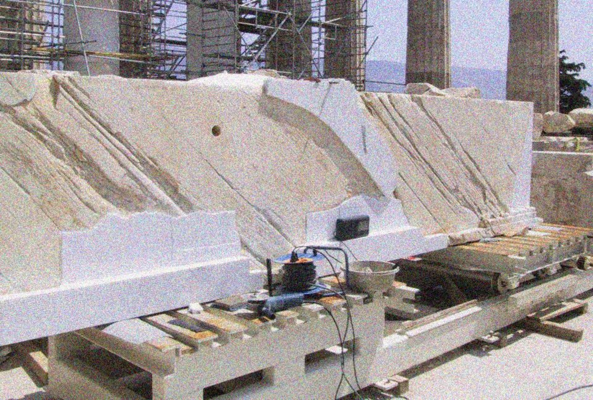
*The assembly of architrave OE.2.1 from its original parts and new marble in the missing areas*
