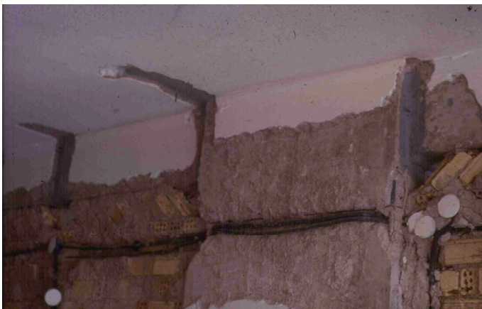
Warning: Supervision does not end with last concrete pour Damage by electrician as no specific path for cables was allowed Note the electric cable pipes are inside the reinforcement!!
