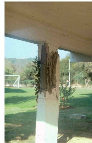
Water drainage pipe in column Not allowed by codes
