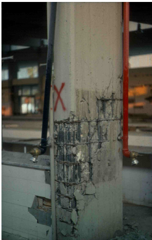
Congestion of reinforced steel bars
