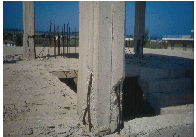
Unacceptable steel bar overlap. Lack of stirrups
