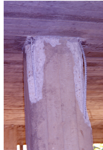
Lack of stirrups
