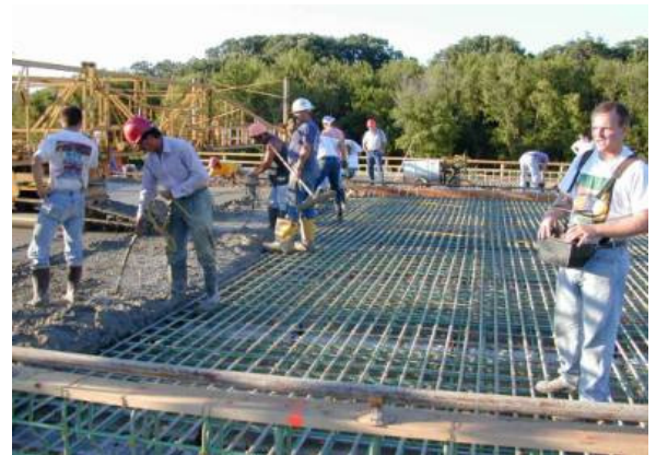
53 rd AVENUE BRIDGE
