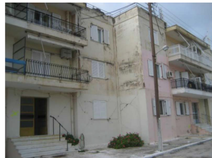
EPPO-ITSAK, 2014. Report on the Mw:6.0 Cephalonia earthquake of 3rd Feb 2014. Earthquake Planning and Protection Organisation-Institute of Engineering Seismology and Earthquake Engineering. http://www.slideshare.net/itsak-eppo/20140203-kefaloniaeq-report-en (downloaded 10/03/14).
