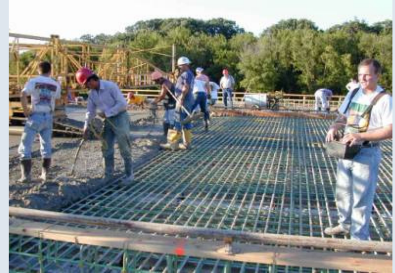
53 rd AVENUE BRIDGE
