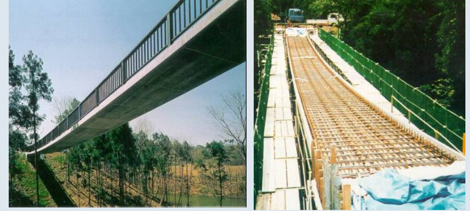
Birdie Bridge - Ibaragi Prefecture, Japan
