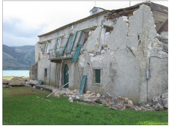
IAS, 2014. Presentation of 2014 Kefalonia earthquakes damage assessment and statistics. Department of Earthquake Recovery, Argostoli, 6th March, 2014
