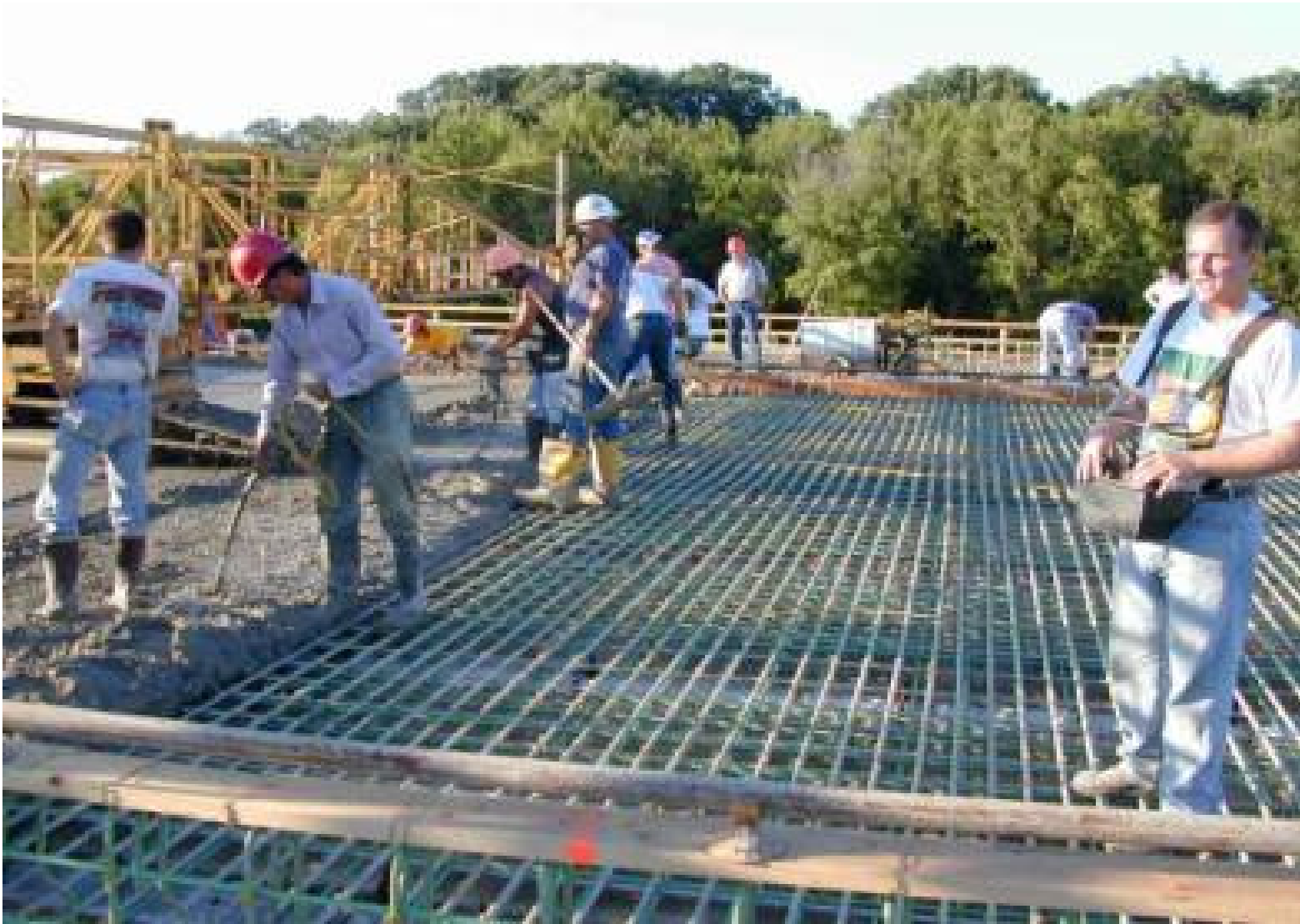
53 rd AVENUE BRIDGE
