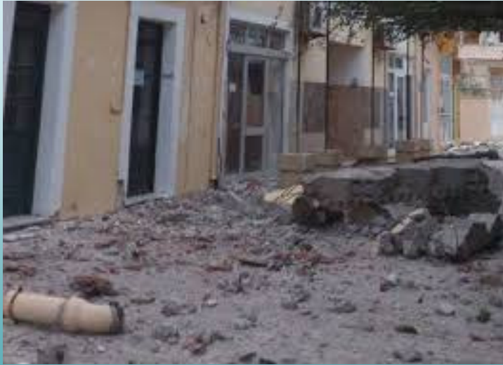
Fatalities can also occur without serious damage to the building
