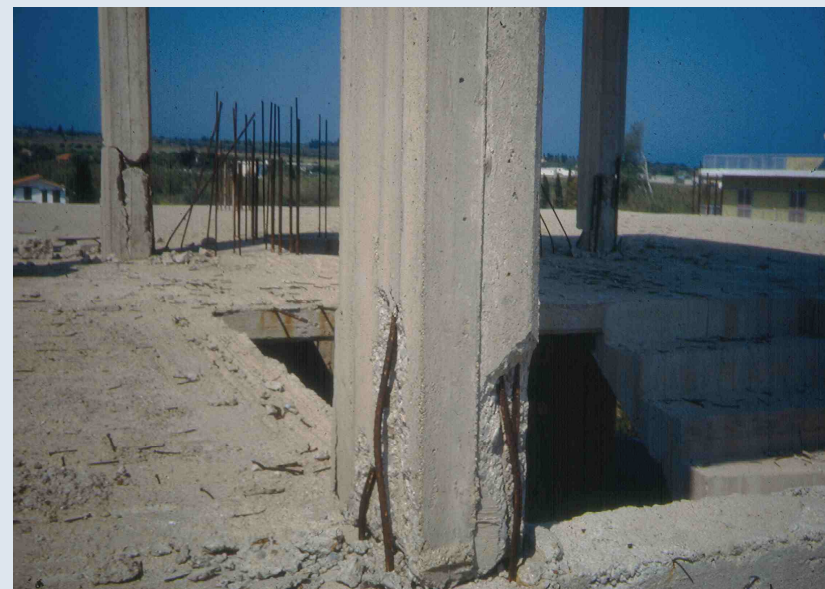
Unacceptable steel bar overlap. Lack of stirrups
