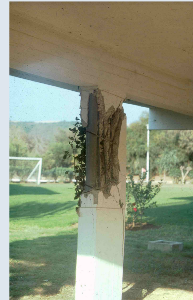
Water drainage pipe in column
