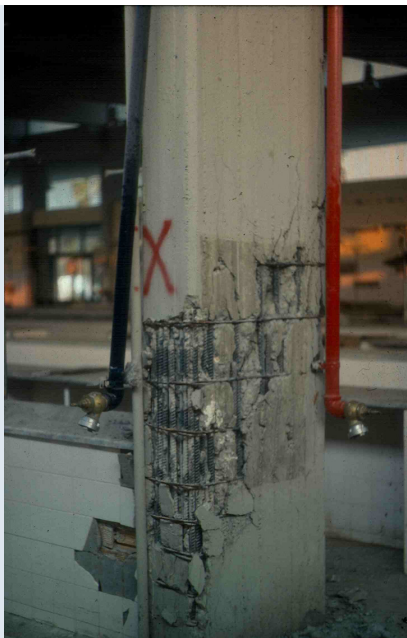
Congestion of reinforced steel bars
