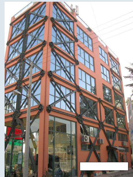
Addition of a bracing system
