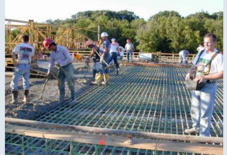
53 rd AVENUE BRIDGE
