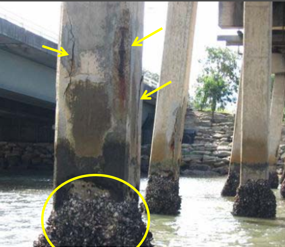
Concrete deterioration of bridge piles
