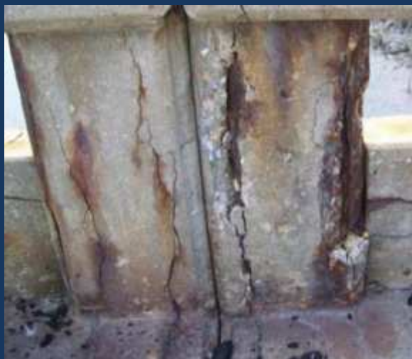
Γέφυρα Deep Creek, USA
