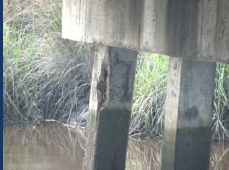
Γέφυρα Riceboro Creek, USA
