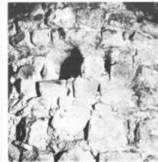
Figure 20.17 Coring, York Minster, England (Courtesy: Shepherd Building Group Ltd.)
