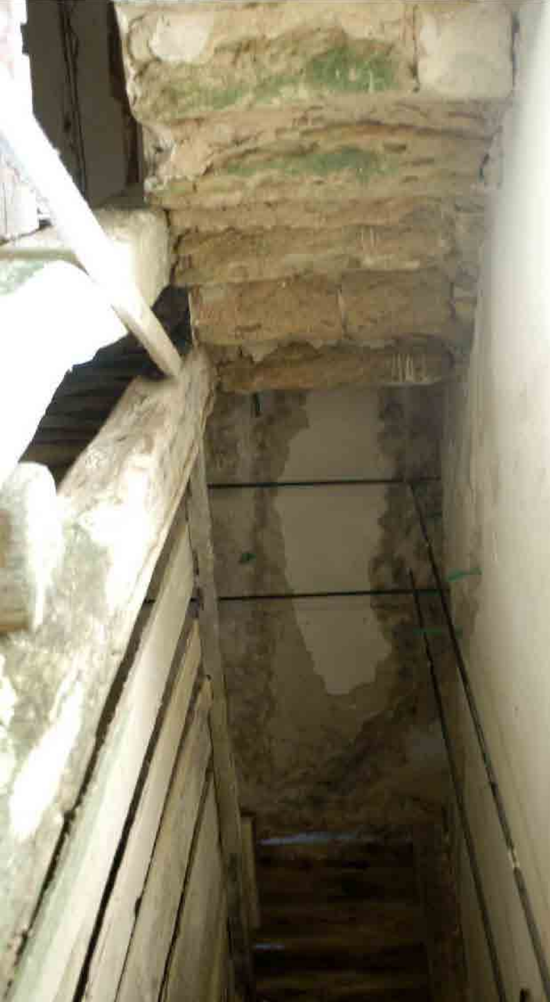
Anchorage with steel \square beam to be adapted inside the building
