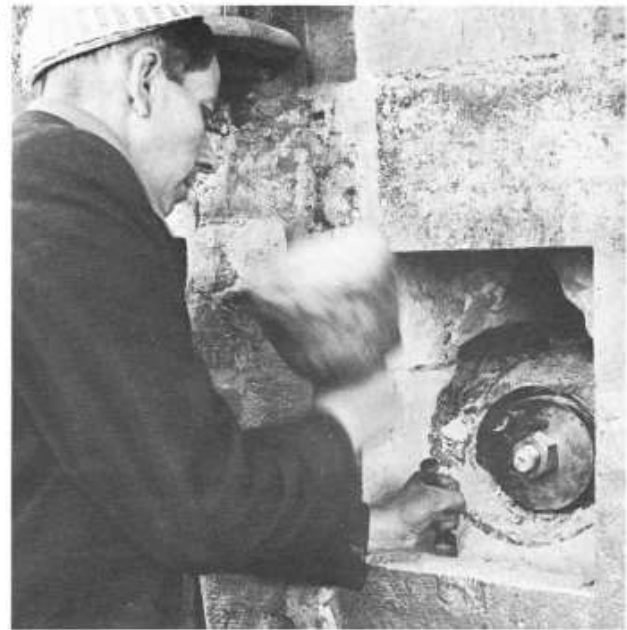
Figure 20.35 Reinforcement, north-west tower, York Minster, England (Courtesy: Shepherd Building Group Ltd)
