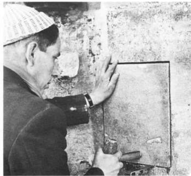
Figure 20.36 Making good, north-west tower, York Minster, England (Courtesy: Shepherd Building Group Ltd)
