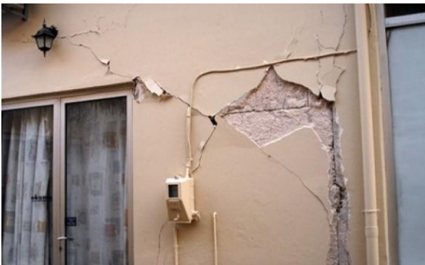
Pic. 1. Damage to masonry ( www.enikos.gr/society )
