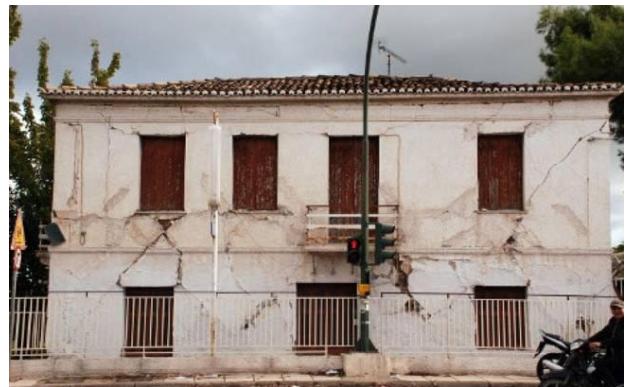
Pic. 2. Structure with differential settlement and minor damage http://www.newsbomb.gr/ellada/news/
